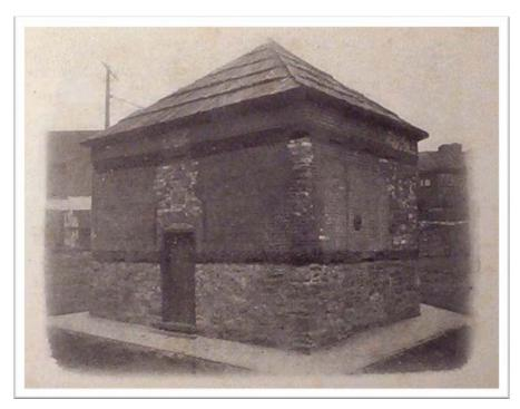
Figure 4. The restored Block House as it appeared in 1902. The variant brick pattern above the door and on the right side of the building mark some areas of repair.
